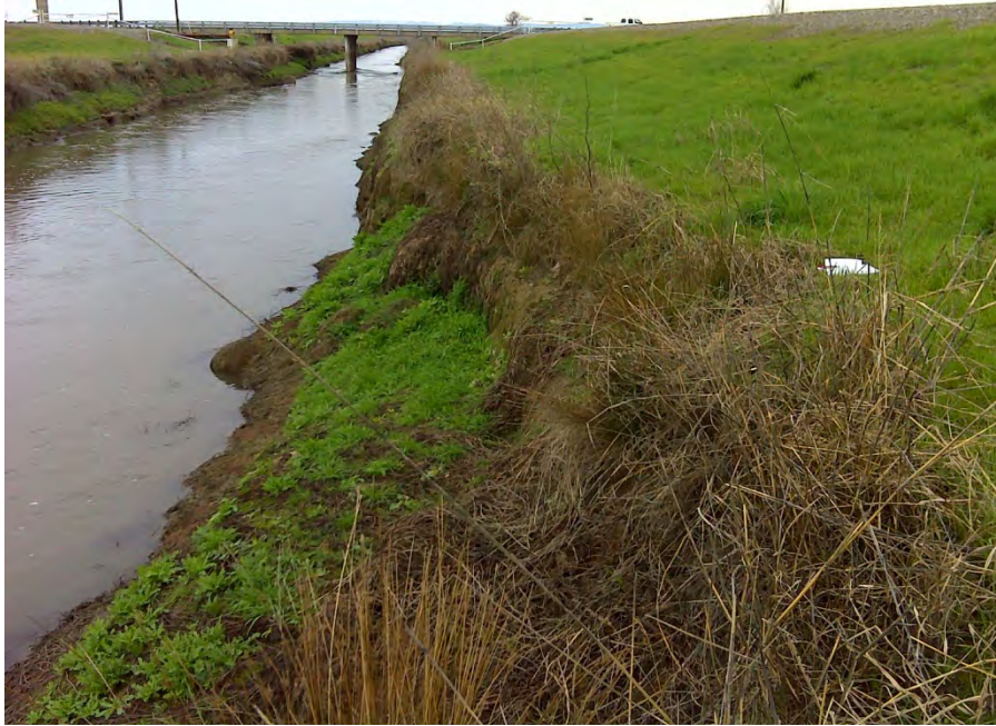
Photo 5. Canal bank erosion, looking upstream.
