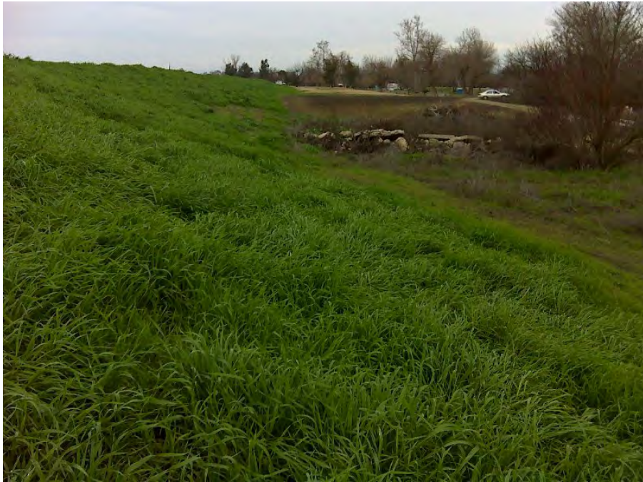
Photo 2. Waterside levee slope, looking upstream.
