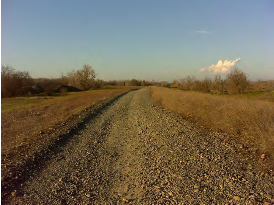
Photo 1. General view of the levee embankment, looking upstream. Feather River channel to the right.
