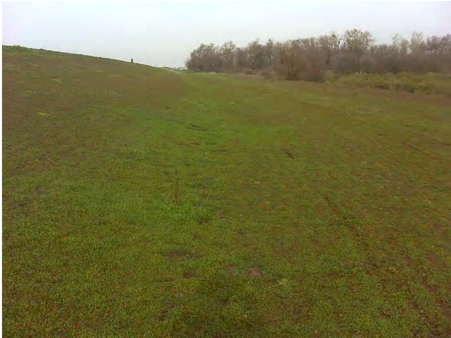
Photo 2. Waterside levee slope, looking upstream.
