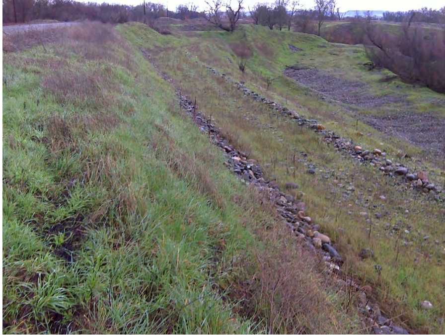
Photo 3. Landside levee slope, looking downstream.
