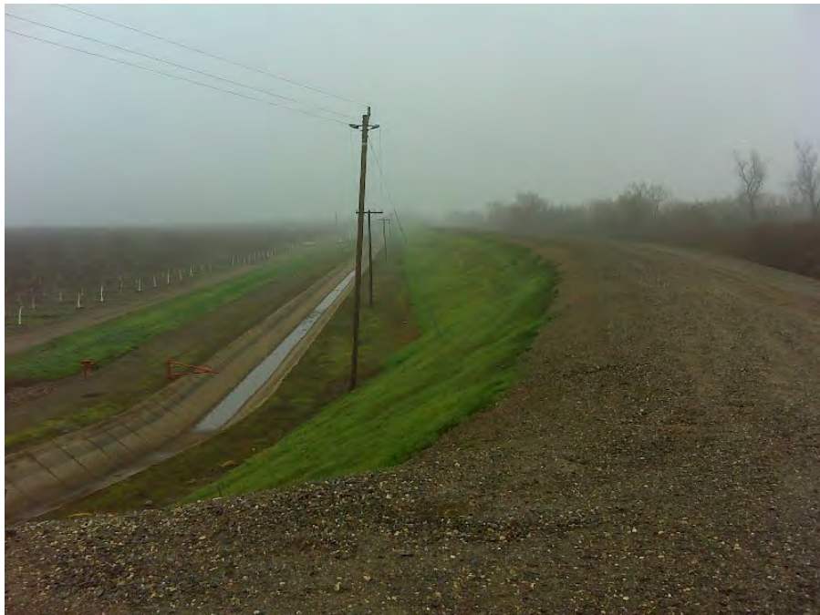
Photo 4. Drainage ditch and power poles near the landside levee toe.
