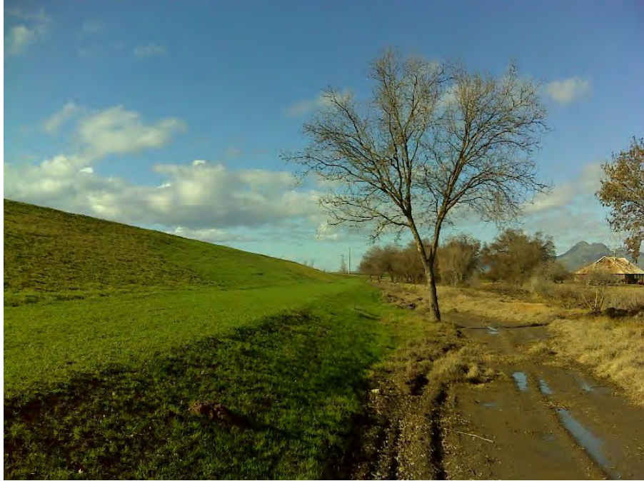
Photo 5. Stability berm at the landside toe, looking upstream
