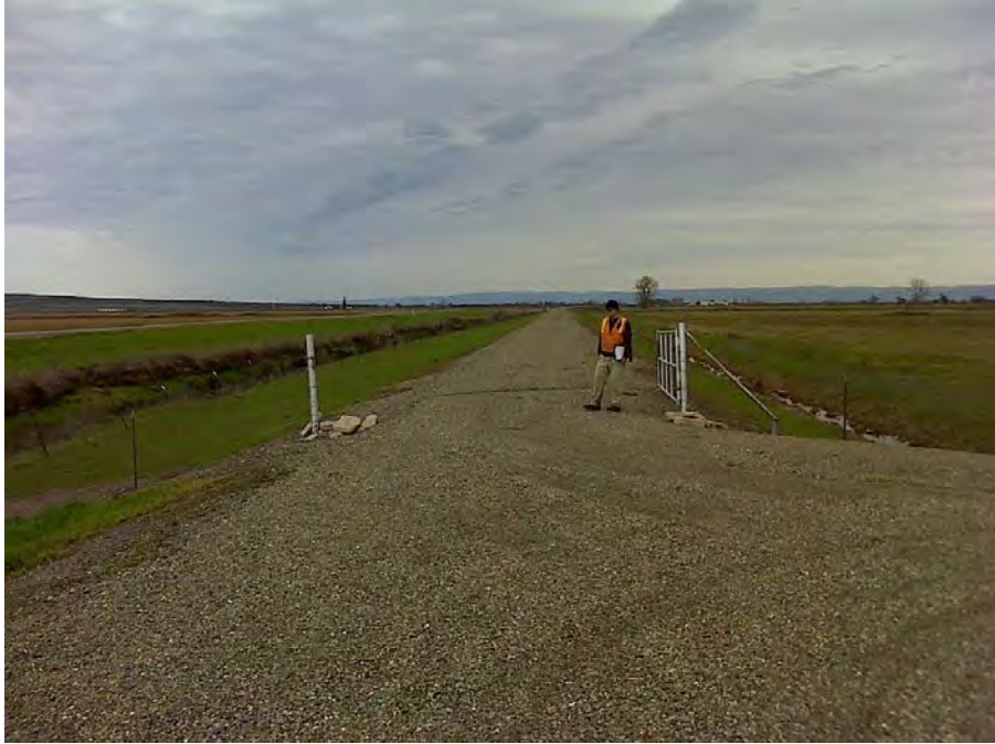
Photo 1. General view of the levee, looking upstream. Canal channel on the left.
