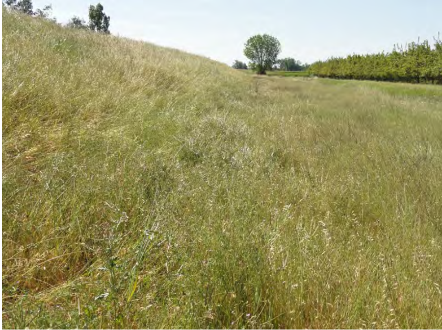
Photo 3. Landside levee slope, looking downstream.
