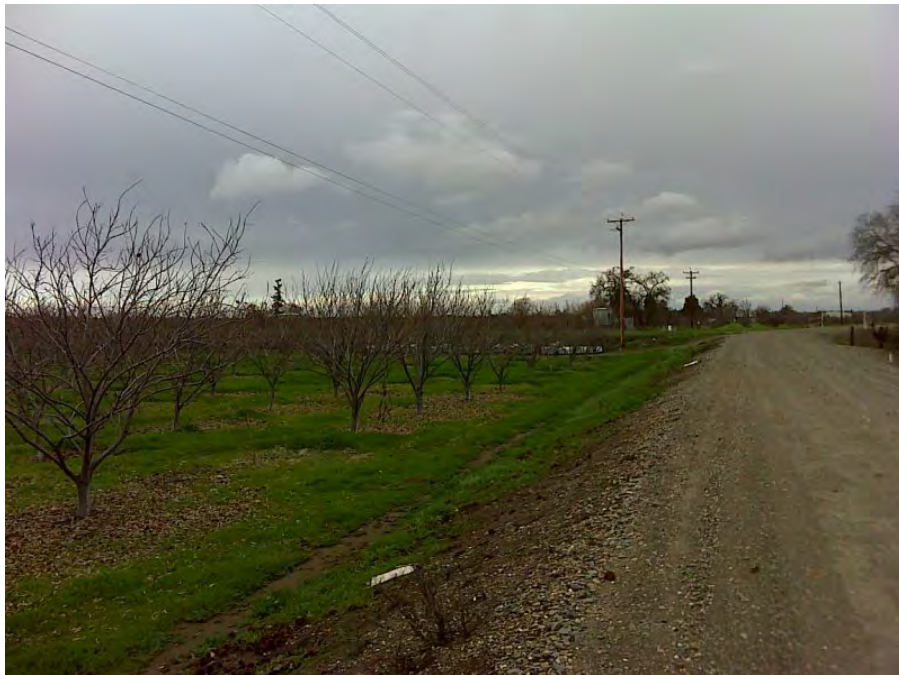
Photo 6. Landside levee slope with powerpoles near the toe, looking upstream.
