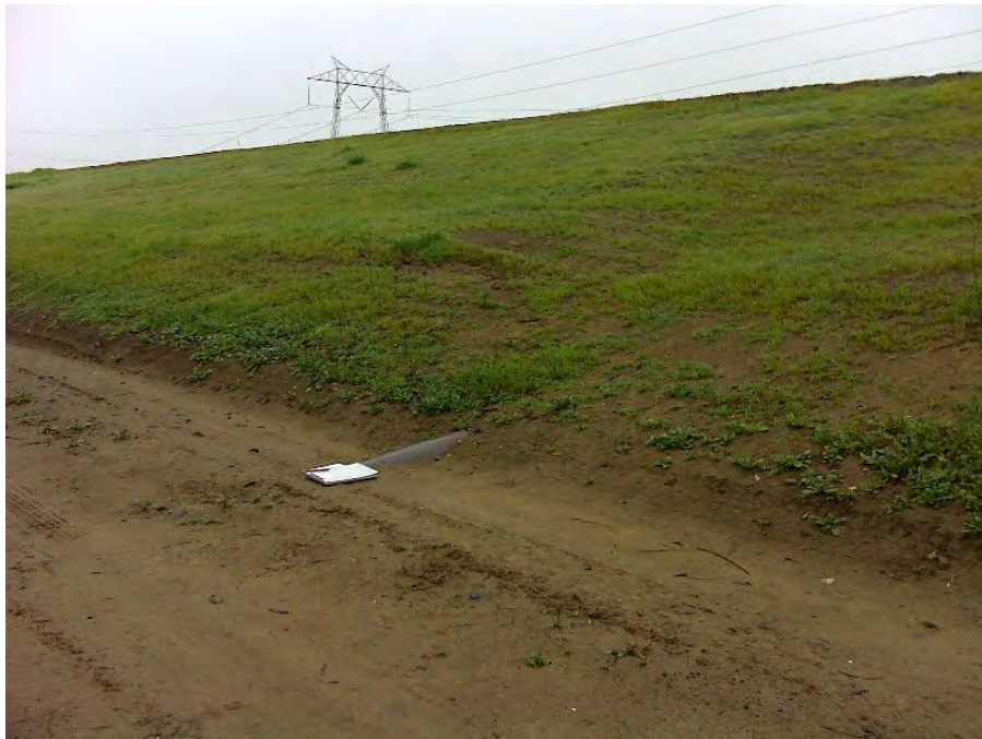
Photo 4. Typical waterside levee slope, looking upstream
