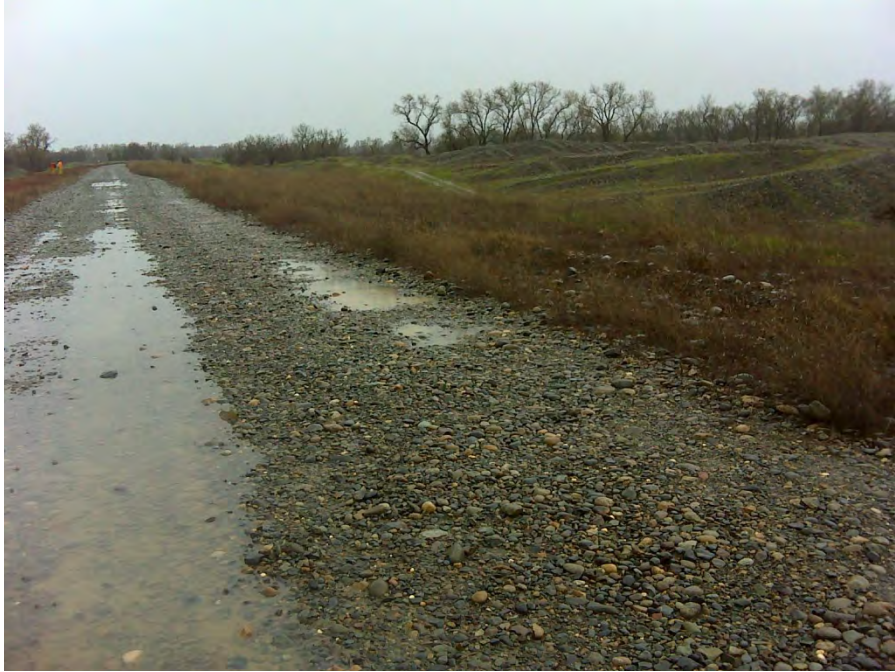
Photo 5. Dredge tailings on the waterside of the levee. Note tailings are higher than the levee crest in some locations.
