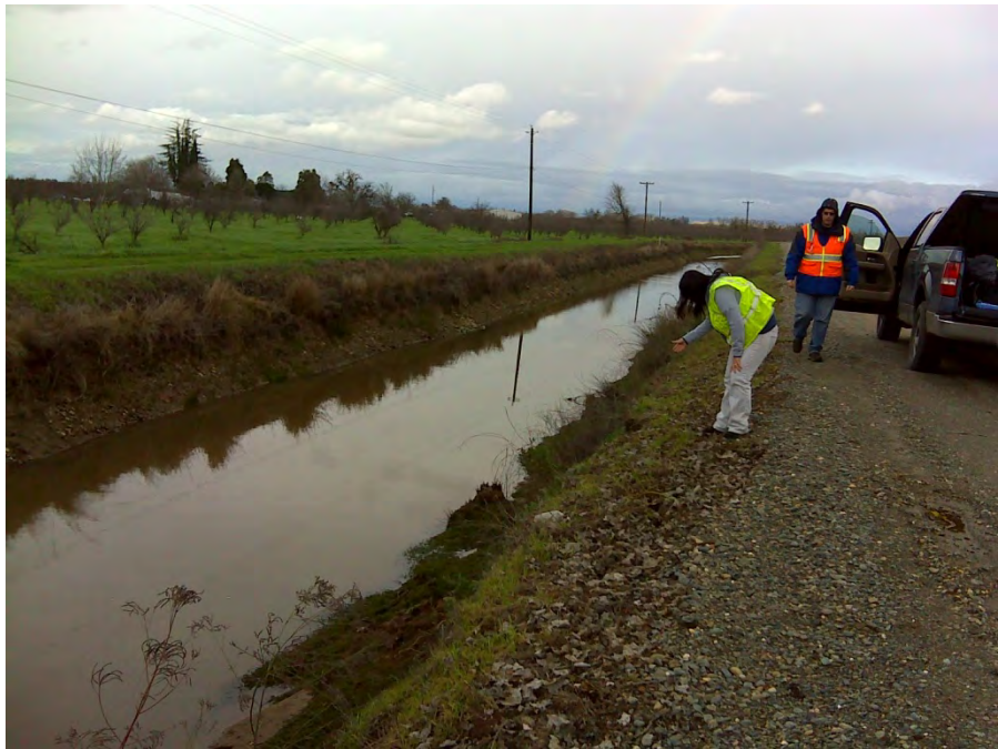
Photo 4. Sutter Butte Canal adjacent to the landside levee toe.
