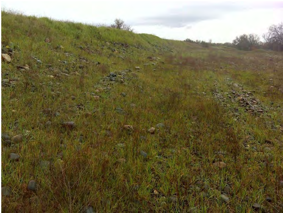
Photo 2. Waterside levee slope, looking upstream.
