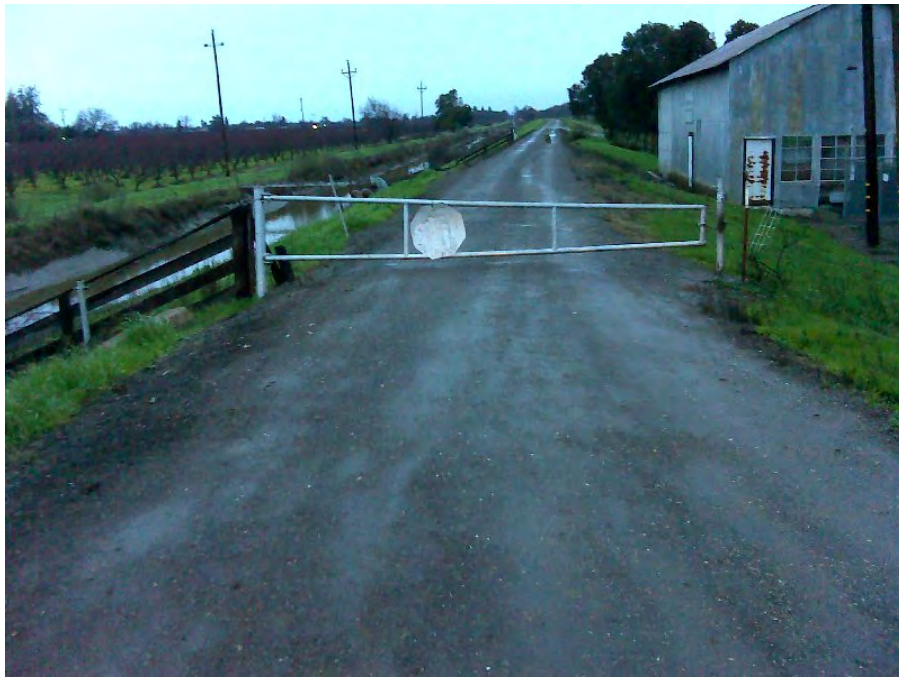
Photo 6. Sutter Butte Canal adjacent to the landside levee toe at the Sunset Pump Plant.
