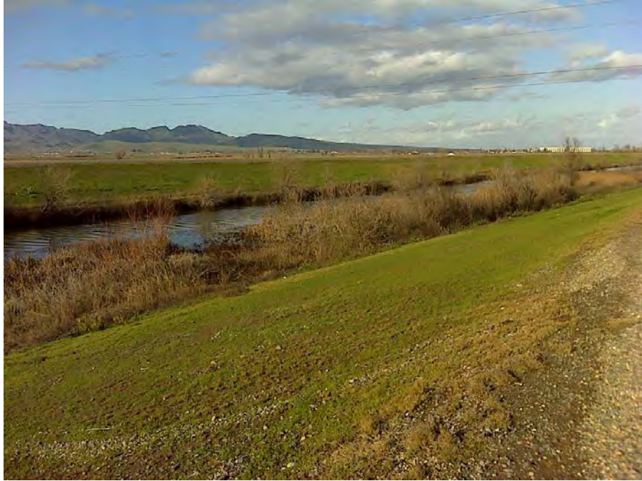
Photo 3. Waterside levee slope and canal, looking north. High ground of Sutter Buttes in the background.
