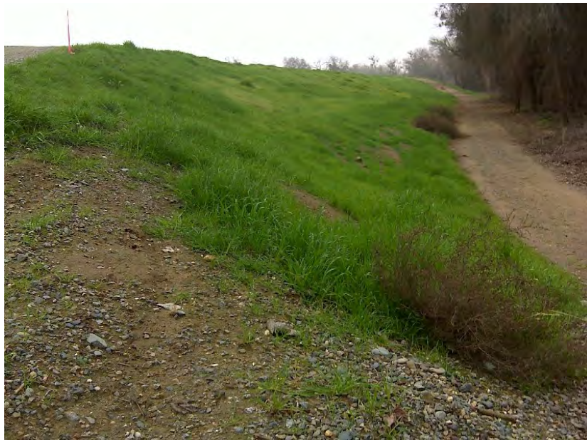
Photo 4. Waterside levee slope, looking upstream.
