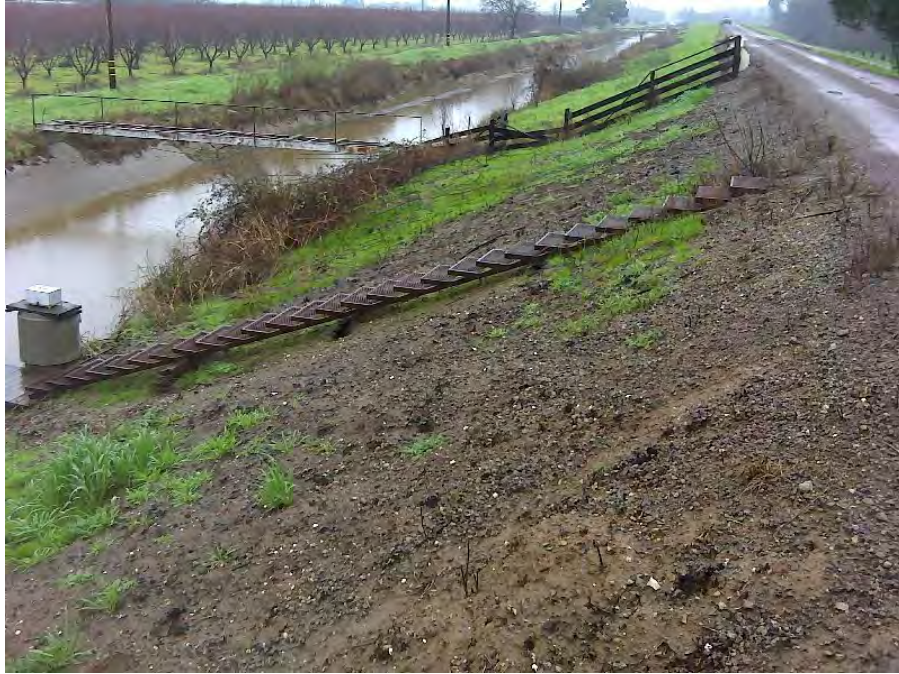
Photo 5. Sutter Butte Canal adjacent to the levee toe.
