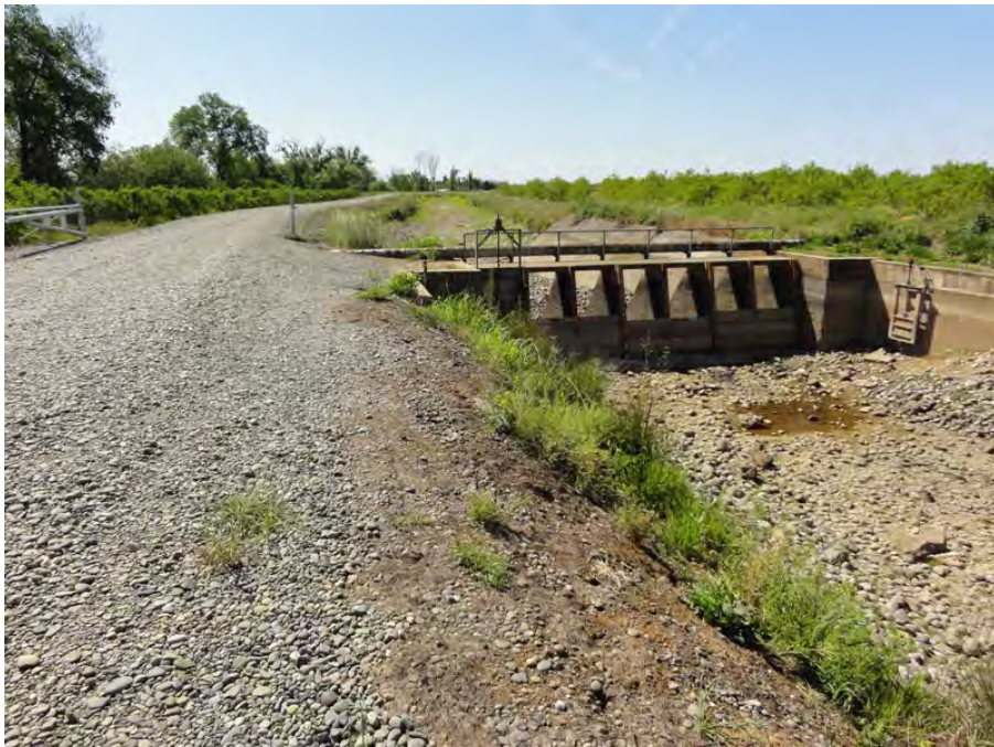
Photo 6. Weir structure in Sutter Butte Canal adjacent to the landside levee toe.
