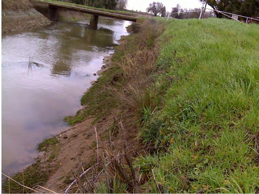
Photo 5. Erosion/sloughing of the landside levee slope into the Sutter Butte Canal.
