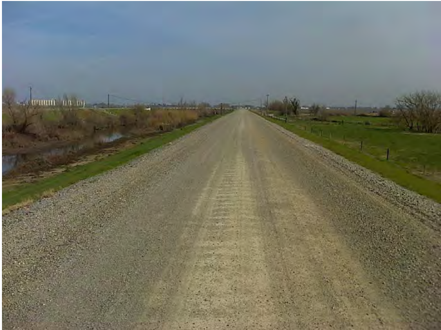
Photo 2. General view of the levee, looking upstream.
