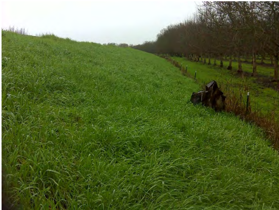
Photo 2. Waterside levee slope, looking upstream.
