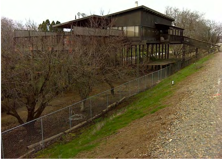
Photo 3. House at the landside levee toe.
