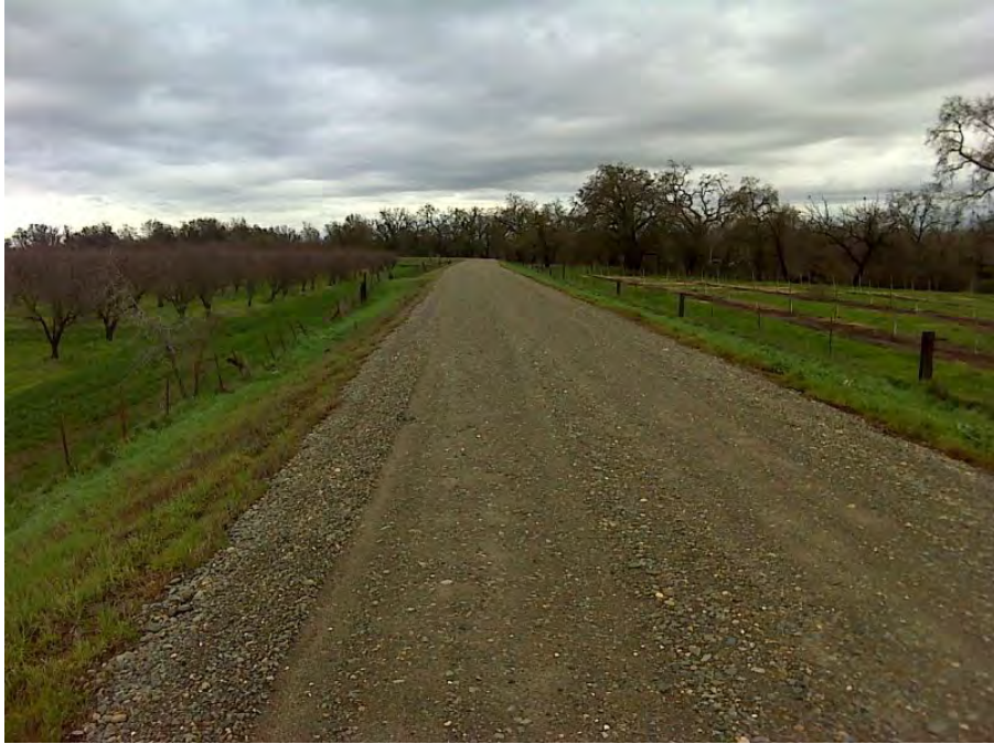
Photo 1. General view of the levee, looking upstream. Feather River channel to the right.
