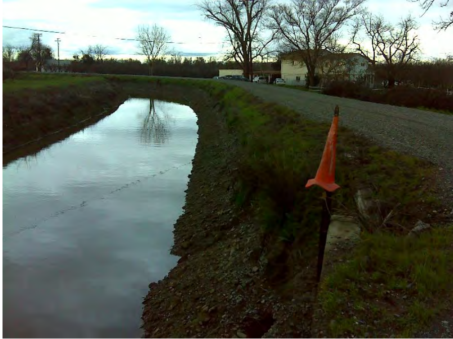
Photo 3. Landside slope erosion/sloughing into the adjacent Sutter Butte Canal; house on waterside of levee.
