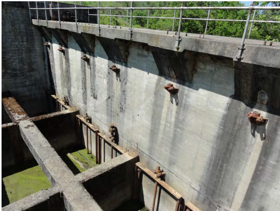
Photo 4. Sutter Butte Canal Headgate Structure. Note gate stems and hoist mechanisms have been removed, leaving the gates “stuck” in the closed position.
