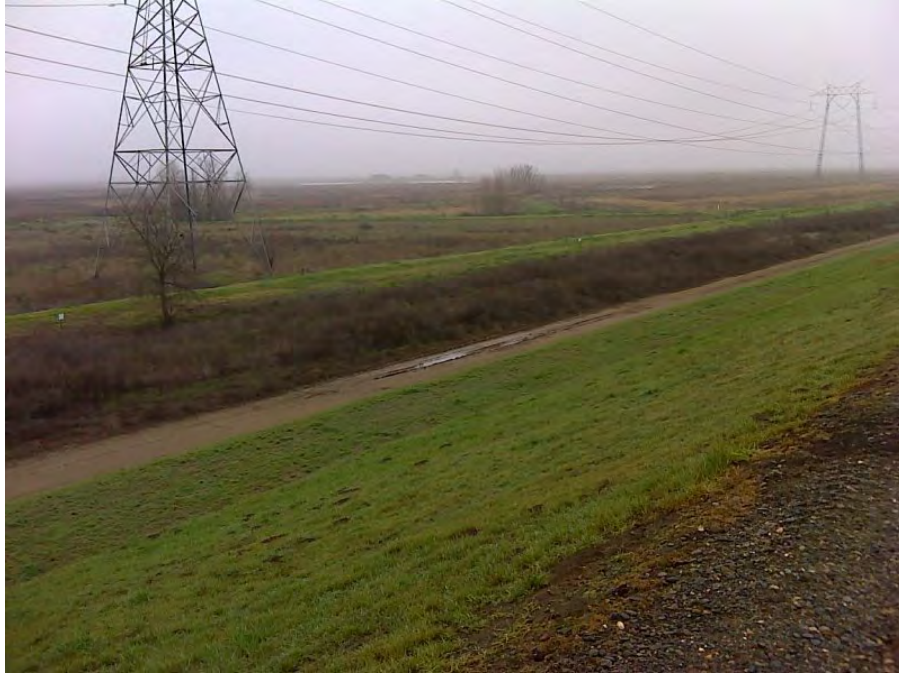
Photo 3 Ditch about 50 feet from the landside toe.
