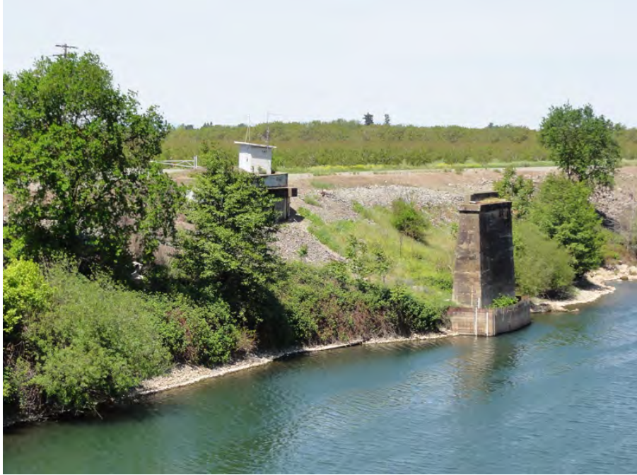
Photo 5. Waterside levee slope at the location of the former Gridley Bridge.
