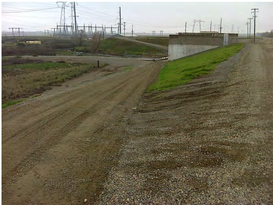
Photo 6. Pump Station No. 2, looking downstream
