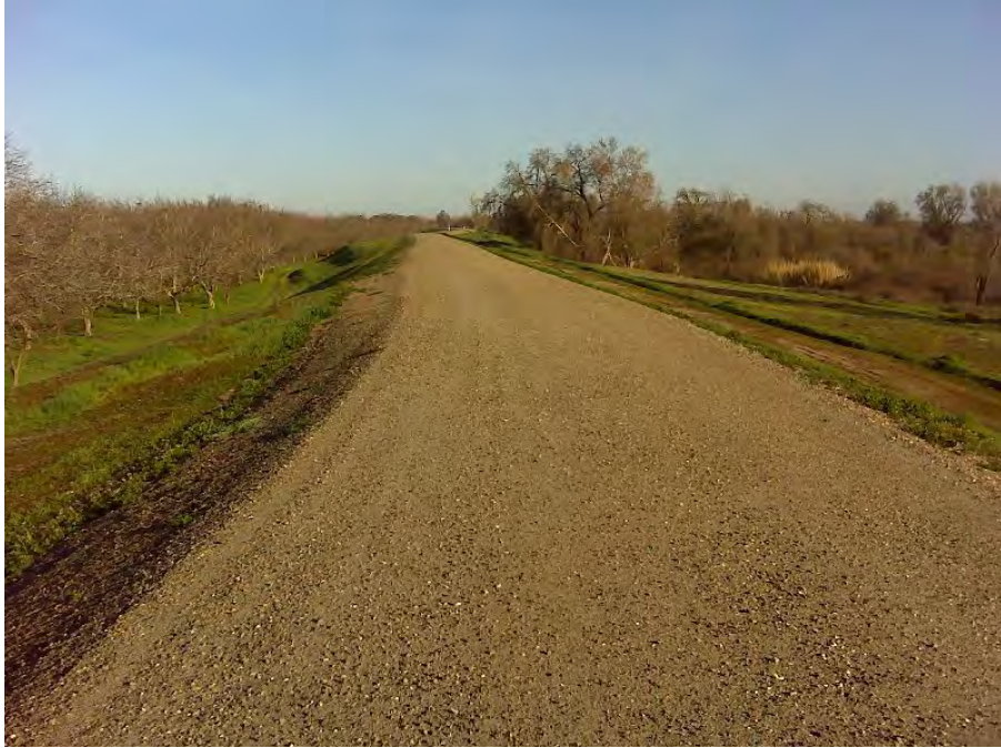
Photo 1. General view of the levee, looking upstream. Feather River channel on the right.
