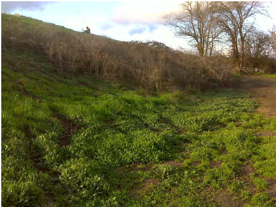
Photo 4. Waterside levee slope, looking upstream.
