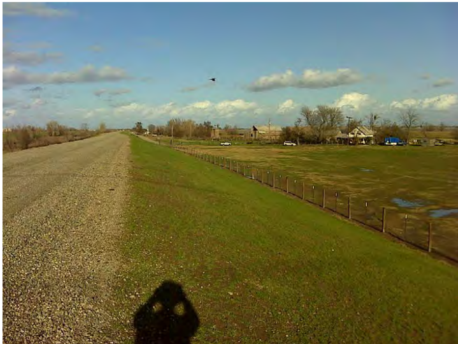
Photo 4. Landside levee slope, looking upstream.
