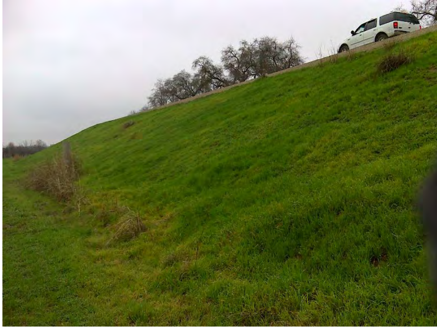
Photo 3. Landside levee slope, looking upstream.
