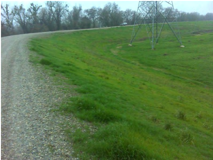
Photo 2. Landside levee slope, looking downstream. Note electrical tower near the toe.
