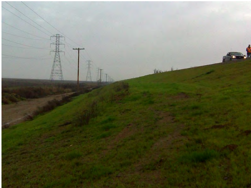
Photo 2. Landside levee slope, looking downstream.
