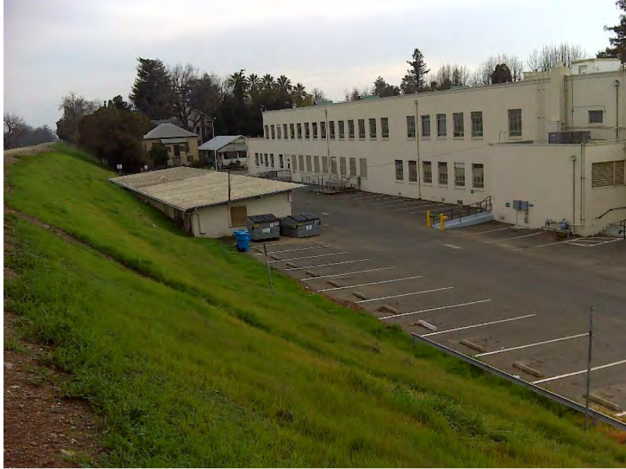
Photo 5. Encroachment into the landside levee slope in Yuba City.
