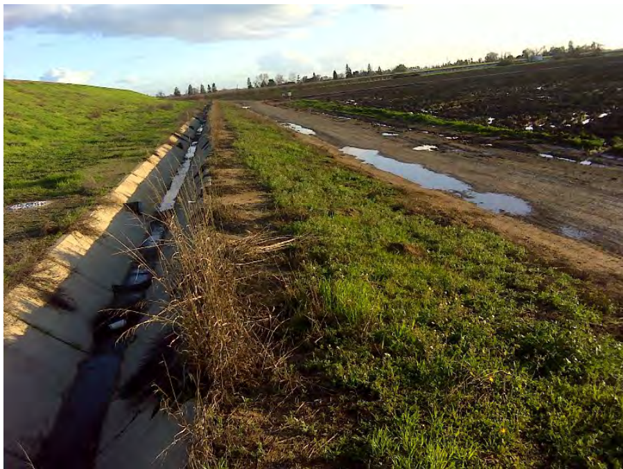
Photo 6. Star Bend relief wells and relief well drainage ditch.
