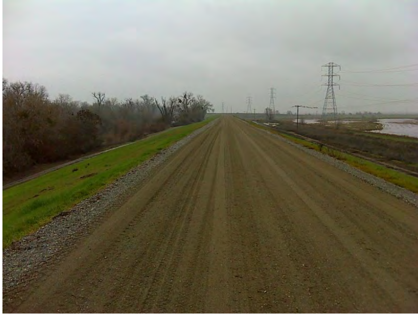
Photo 1. General view of the levee, looking upstream. Bypass channel is on the left
