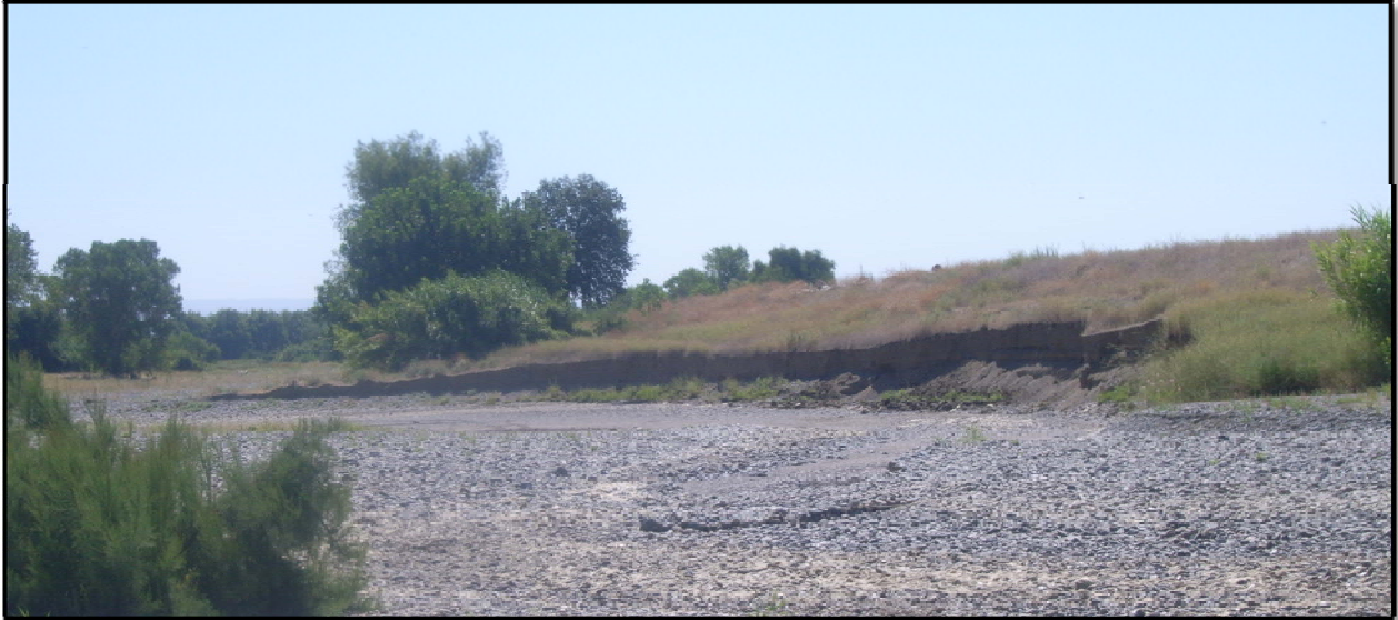
Figure 20. Typical View of the Channel and Eroding Bank of Elder Creek.
