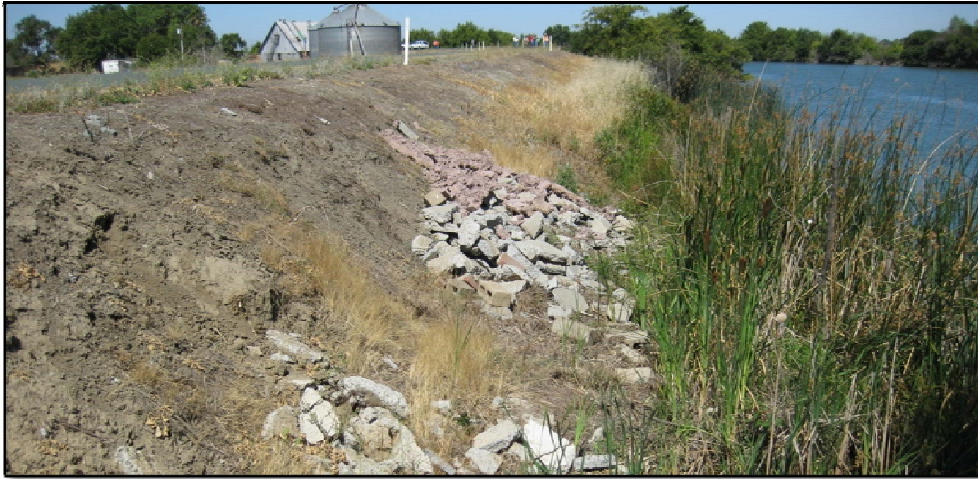
Figure 11. Typical View of Georgiana Slough.
