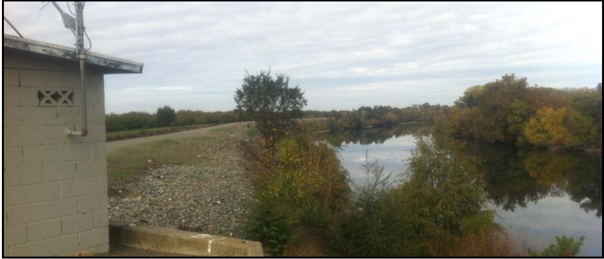
Figure 14. Typical View of the Northern Reach of the Feather River.
