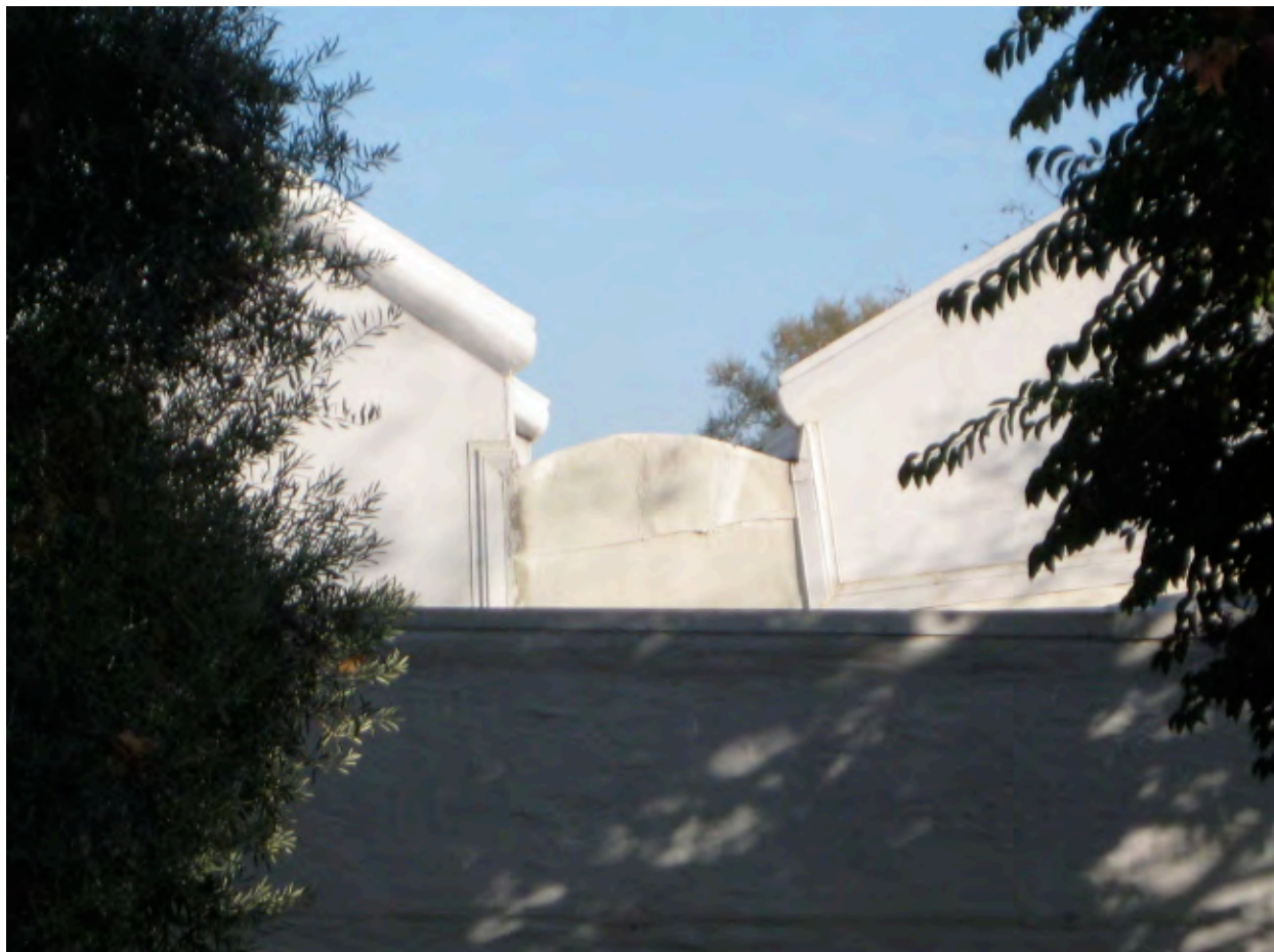
Figure 5. Horizontal crack in barrel vault. Even though the roof was repaired and strengthened in 2006, horizontal cracking in the small barrel vaulted section is ongoing. (Photo by Garavaglia Architecture, Inc., 2011.)
