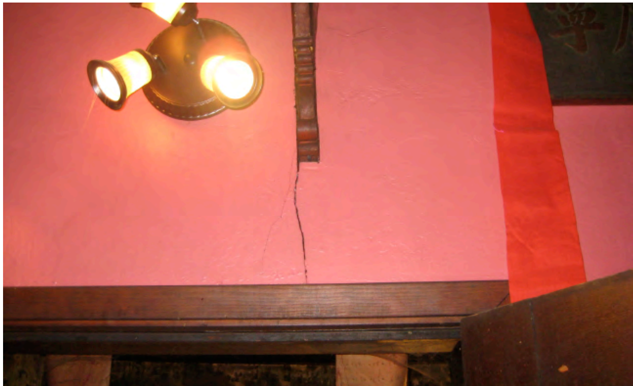
Figure 6. Crack in the new wall paneling. This crack is above the door to the Fortune Readers's Room. The condition of the underlying brick wall could not be surveyed. (Photo by Garavaglia Architecture, Inc., 2011.)
