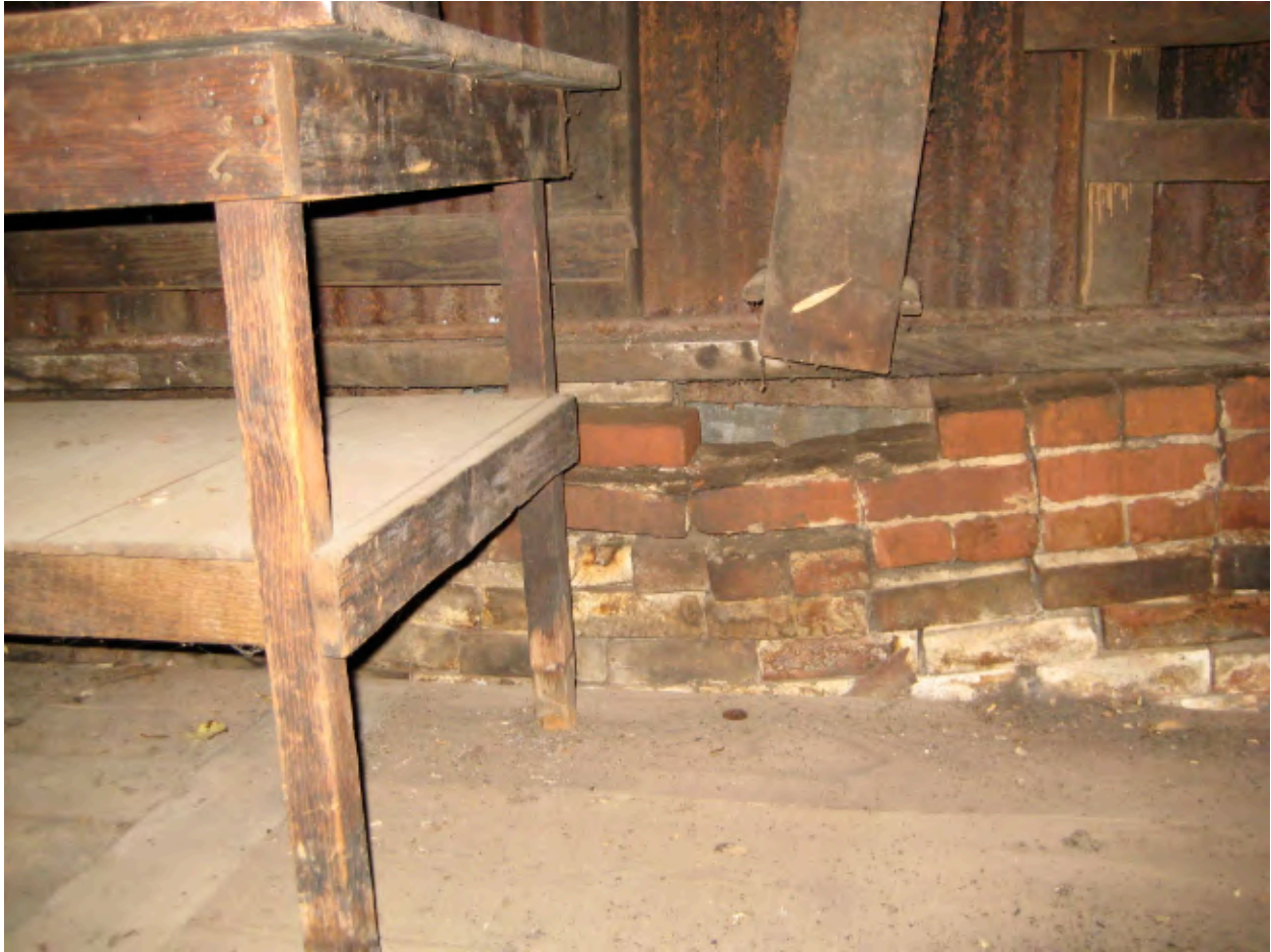
Figure 8. Poor pony wall condition. The northeast corner of the Temple is wood frame on a brick pony wall. The framing and the masonry wall are in poor condition. This image shows one area of extreme damage where severe settlement has occurred. (Photo by Garavaglia Architecture, Inc., 2011.)
