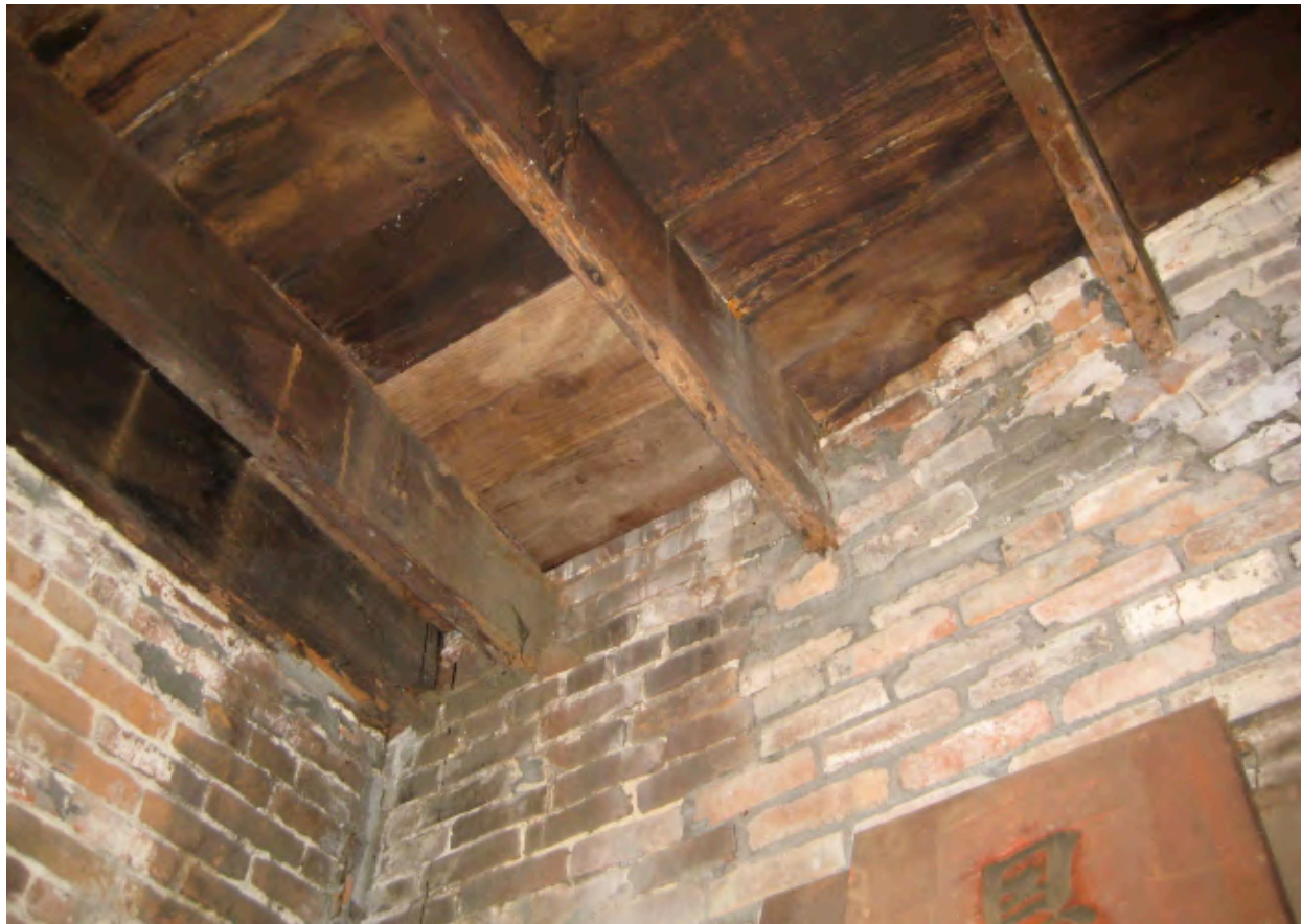
Figure 7. Moisture staining in the Gambler's Room. This area is near a roof drain that was improperly functioning. The area has since been repaired, but the damage is evident. (Photo by Garavaglia Architecture, Inc., 2011.)
