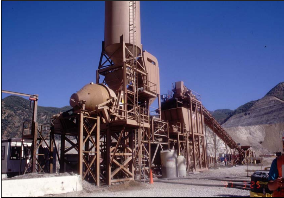
Photo 1. Typical Batch Plant Operation
