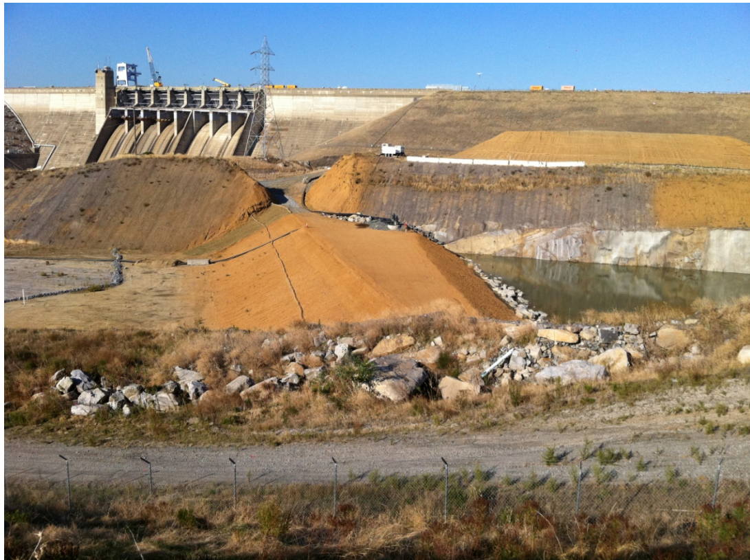
Photo 2. Dirt Access Road Location
