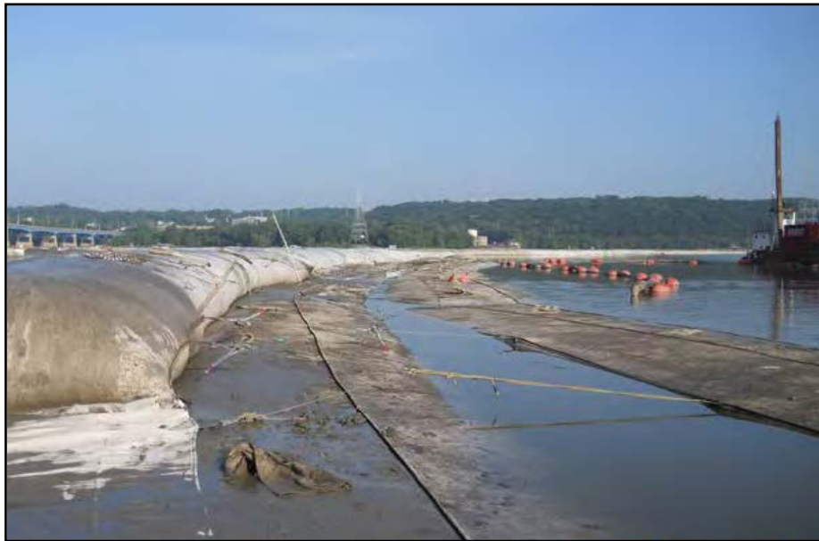
Photograph 5. Island Construction Using Geotextile Containers, Illinois Waterway near Peoria, Il.
