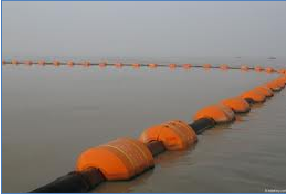
Photograph 3. Floating Dredge Material Transport Pipeline
