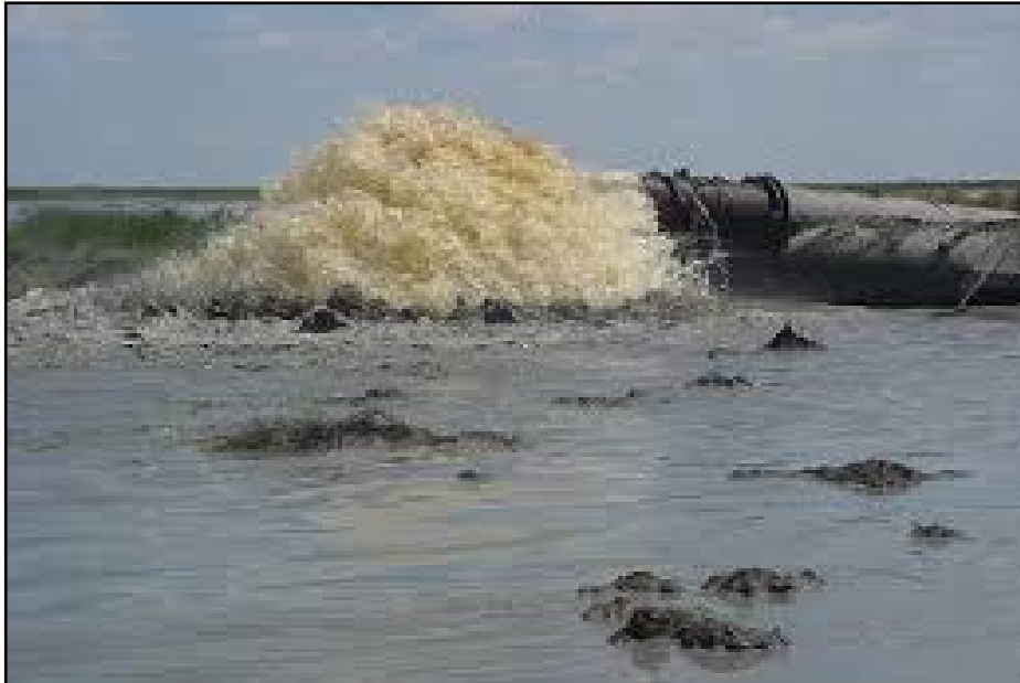
Photograph 4. Slurry Outfall
