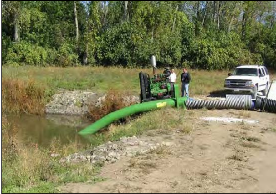
Photograph 1. Portable Water Pumping System
